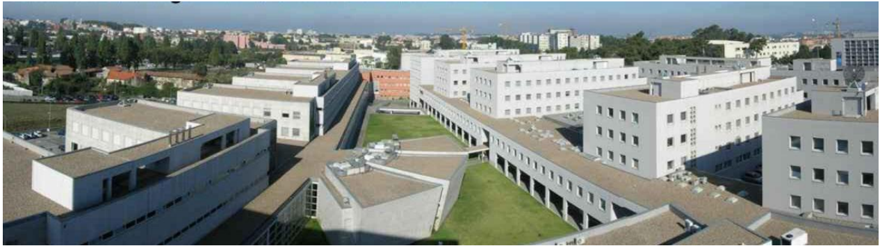
Figure 3.2 - Panoramic view of campus from the Library building
